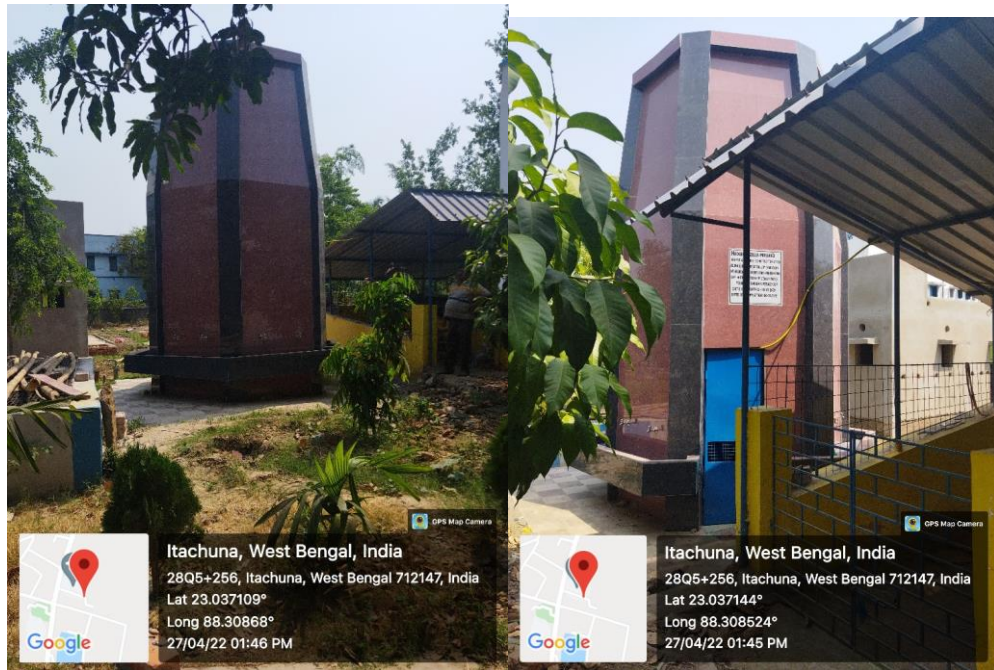
Water reservoir with bore well system
